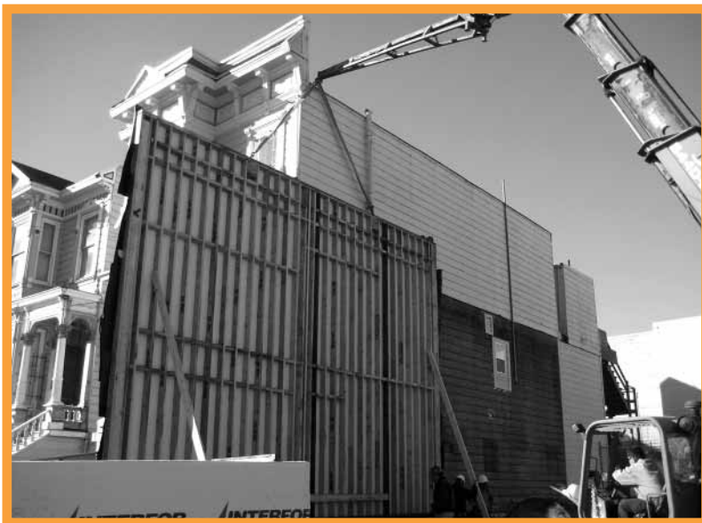
February 2008 — builders lift the South wall into place.
