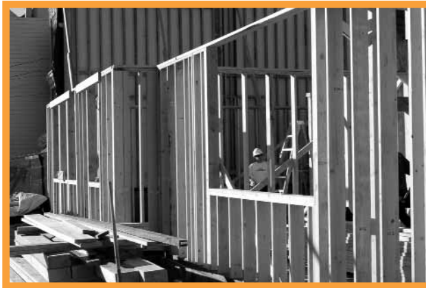
February 2008 — the first floor of the East wall, on Baker Street.
