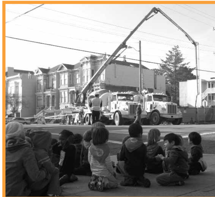
January 2008 — students watch cement mixers pouring the foundation.
